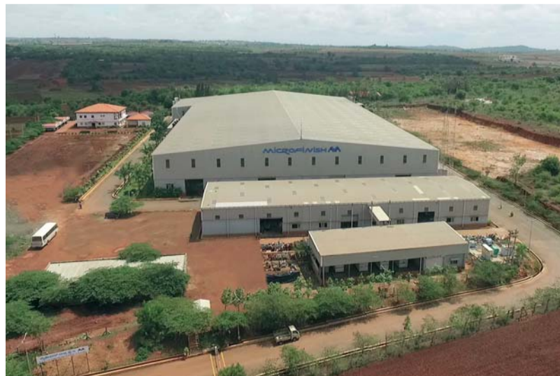
An aerial overview of the Itigatti facility.
